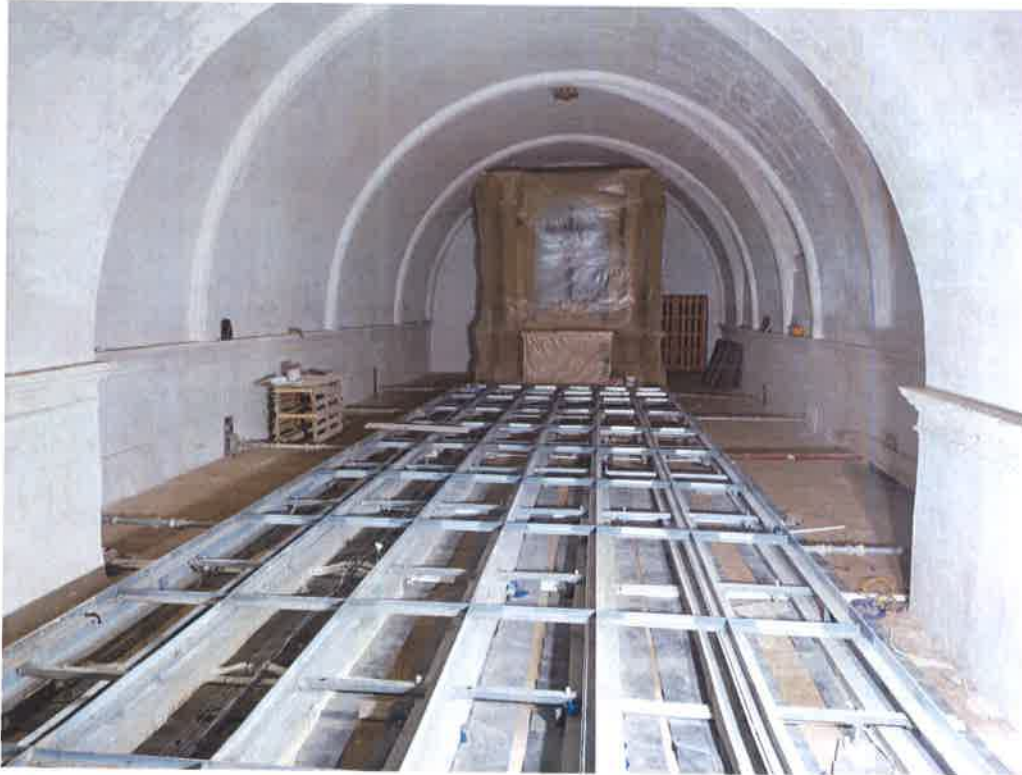
Photograph taken by the Commissioner during the site inspection.
